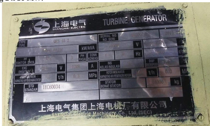
Gambar 1. Name Plate Generator PLTU Bengkayang 2 x 50 MW
