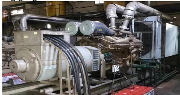
Gambar 1. mesin diesel Cummins KTA 38-G5.
