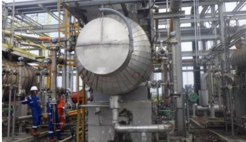
Gambar 1. High Pressure separator (D-0101)
